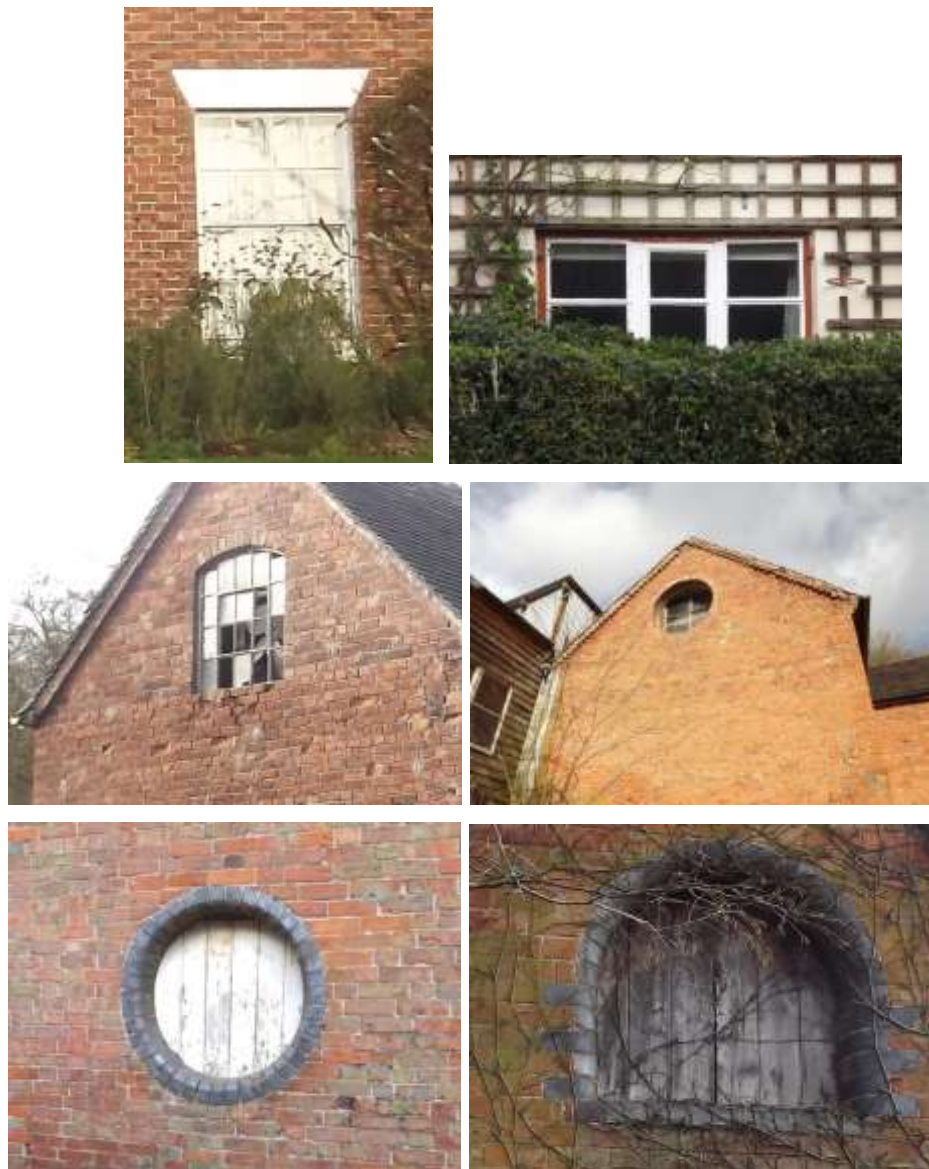
Figure 10 A variety of window openings and styles can be found within the Conservation Area
