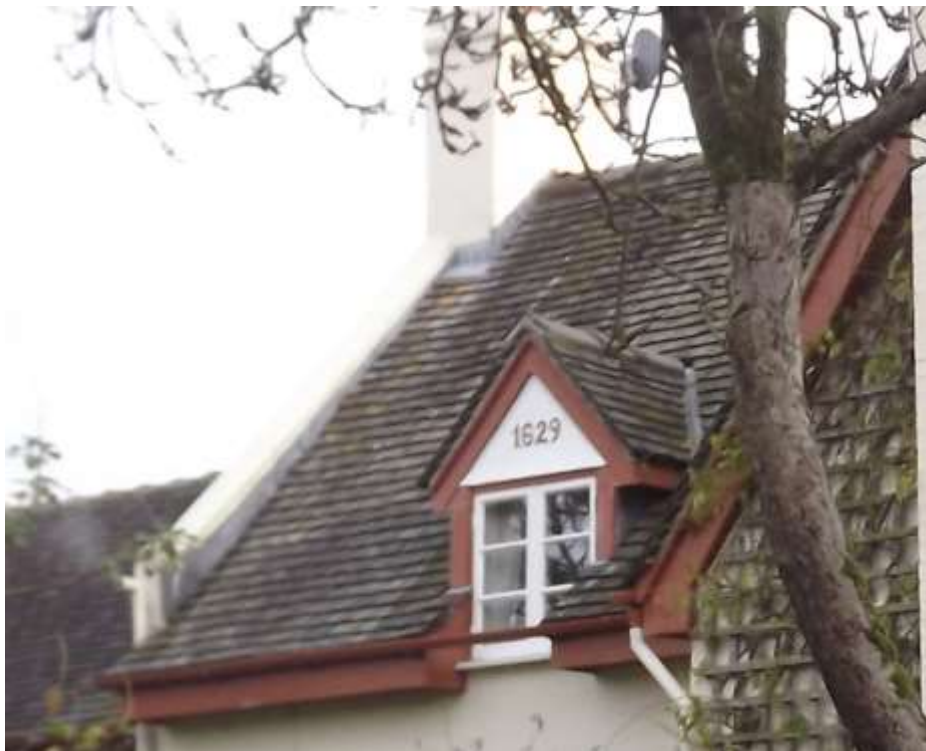
Figure 9 Gabled dormers to the roof of The Cottage
