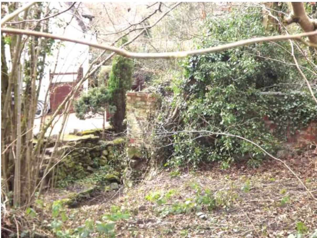
Figure 36 Brick and stone walling to the demolished smithy
