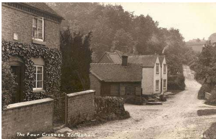
Figure 1 Historic photograph from between 1915-1930, showing the now demolished smithy and the Four Crosses (now Brook House) beyond. Greatwood Cottage can be seen in the foreground.
