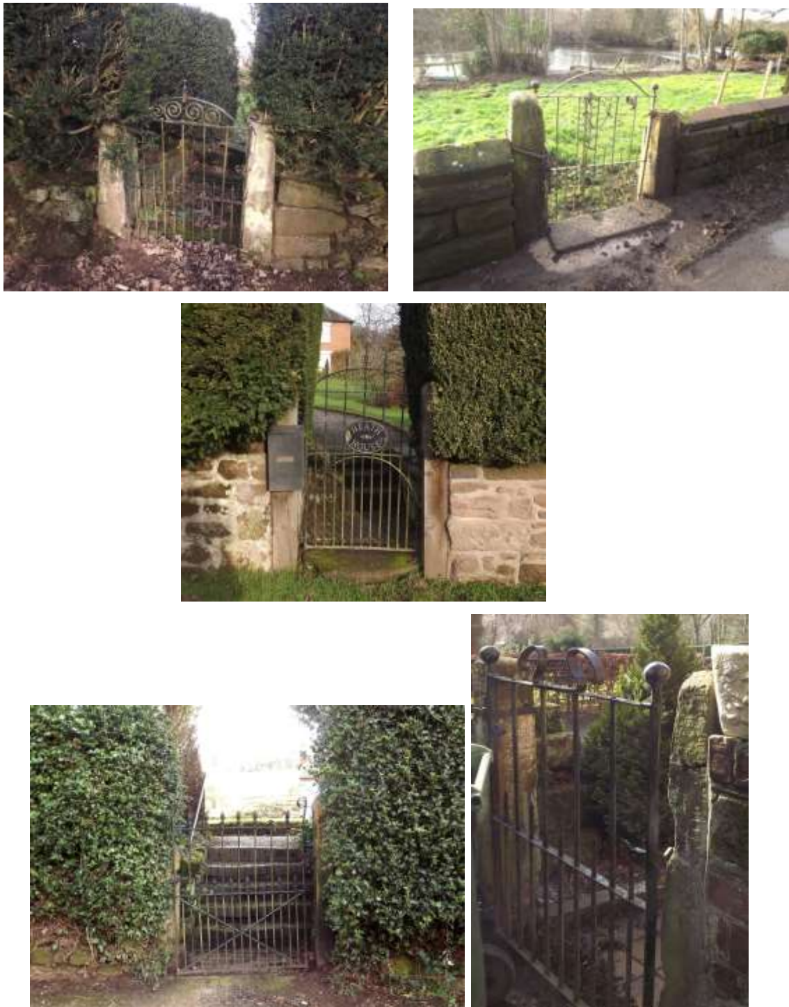
Figure 13 Wrought iron gates add architectural interest to the Conservation Area
