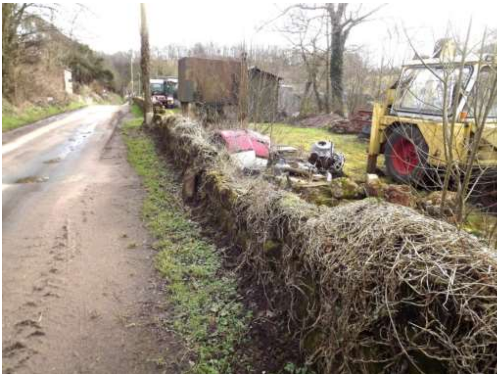
Figure 39 Some important boundary walls have fallen down or are hidden behind overgrown hedgerows.
