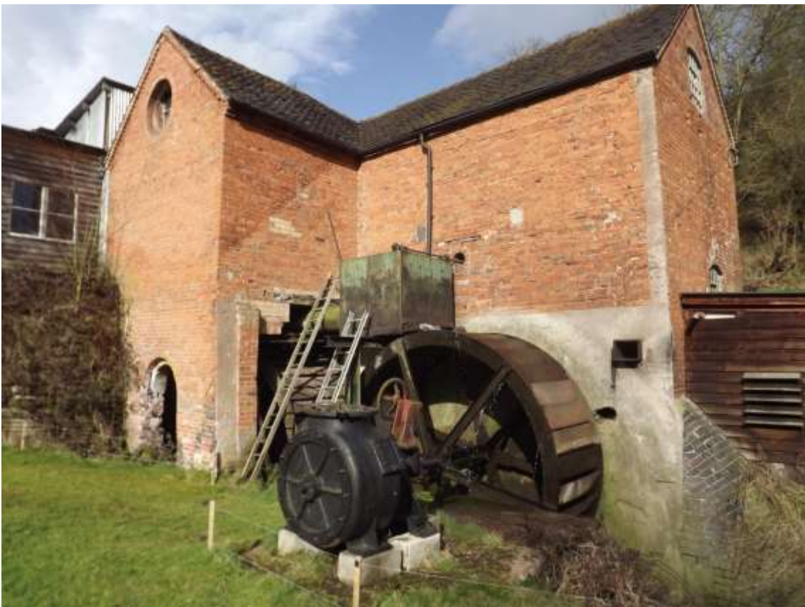
Figure 25 Waterwheels to the rear of the mill building
